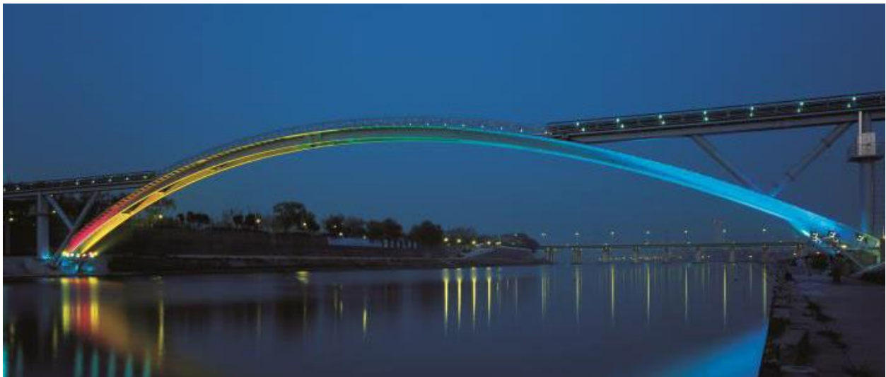
Figure 2: View of the Seonyu “Footbridge of Peace” in South Korea (Lafarge, 2009)
