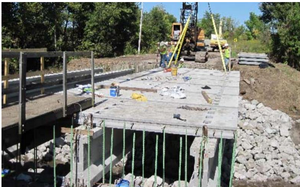
Figure 10: Setting the UHPC Waffle Deck panels (Heimenn, 2013)
