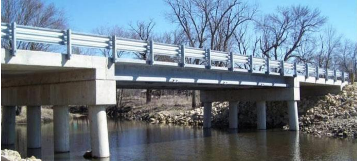
Figure 5: Picture of the Jakway Bridge (FHWA, 2013)
