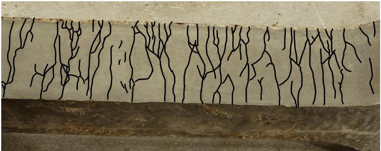
Figure 47: Micro-cracking in Supplier 1 - 2% Fiber Specimen - with marks
