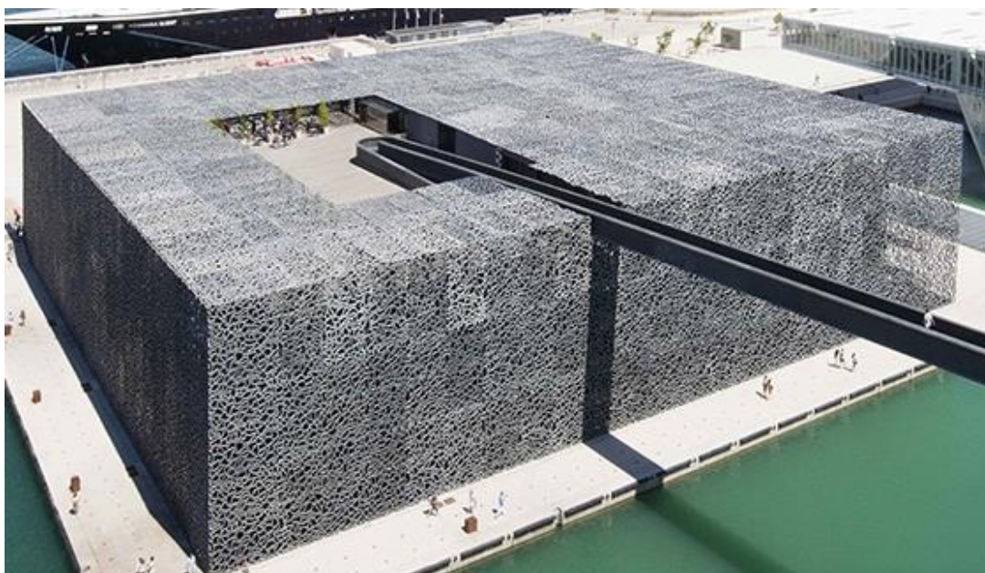
Figure 14: UHPC lattice facade and footbridge MUCEM (Photo by Rudy Ricciotti)
