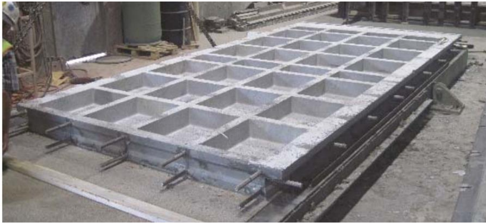
Figure 9: UHPC waffle deck panel with formwork removed - panel upside down (Heimenn, 2013)
