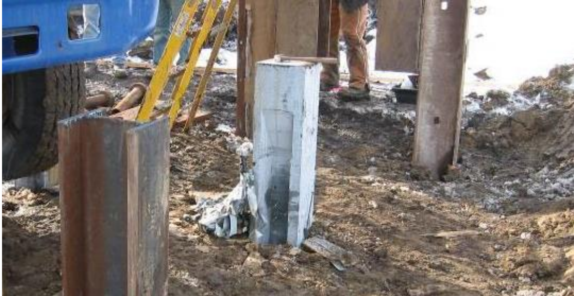
Figure 8: Experimental precast pile made of UHPC (Source: Iowa State University)
