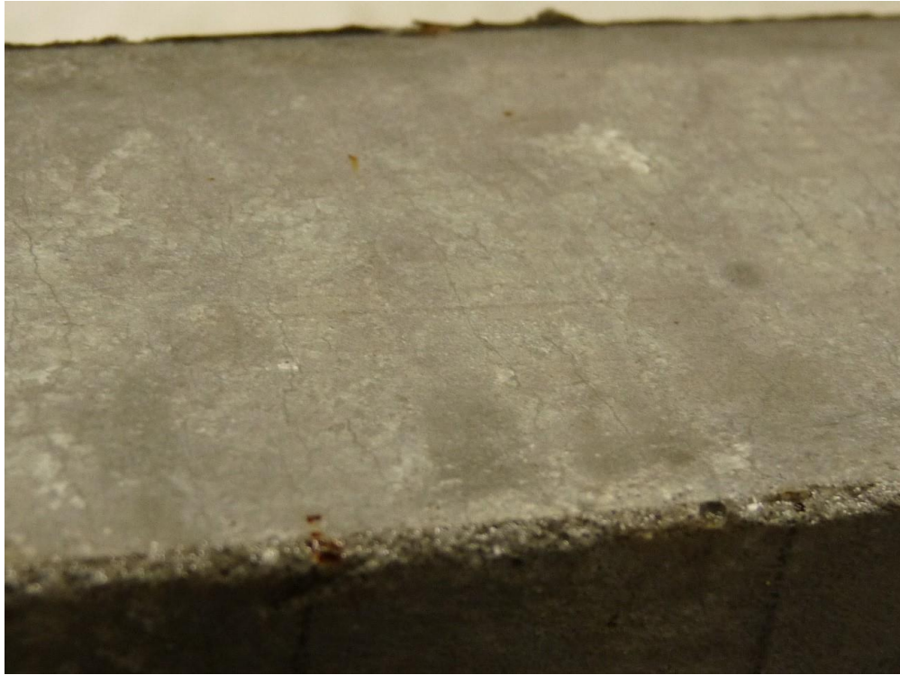
Figure 48: Micro-cracking in Supplier 1 - 1% Fiber Specimen
