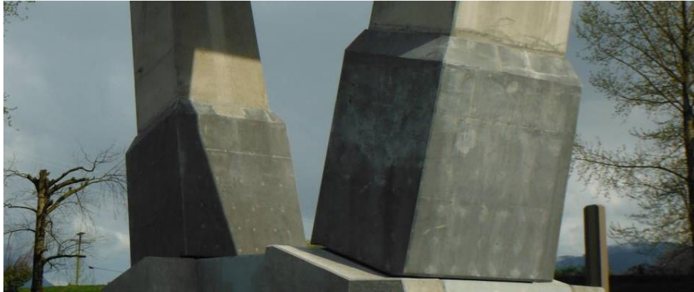
Figure 11: Picture of finished Mission Bridge pier jacketing (Source: Ductal)
