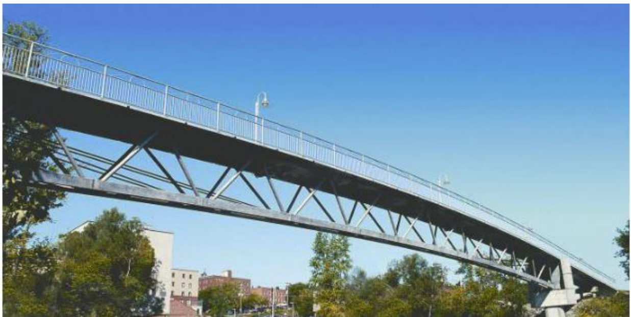
Figure 1: View of the finished Sherbrooke Pedestrian Bridge (FHWA, 2013)
