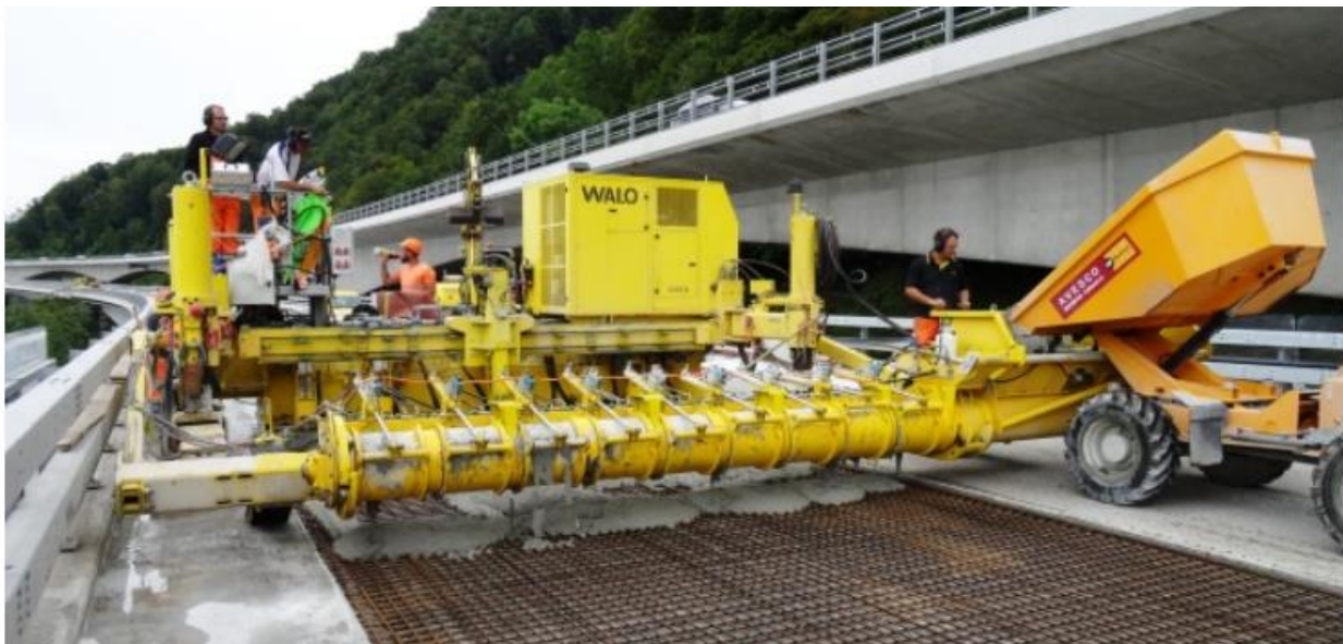
Figure 7: Construction being performed on the Chillon Viaducts (Source: Ductal)
