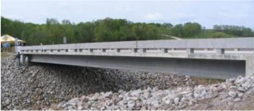
Figure 4; Photo of the completed Mars Hill Bridge (FHWA, 2013)
